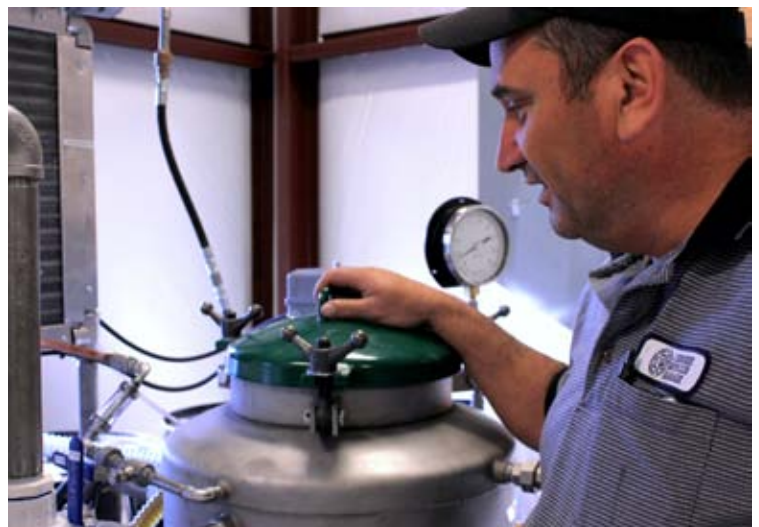
Donnie Owle, Shop Manager, inspects the biodiesel equipment. The CBC Biodiesel Program can make 250 gallons of fuel per day. Used cooking oil for the program is collected from local businesses. All of the Club's school buses run on this alternative fuel.
